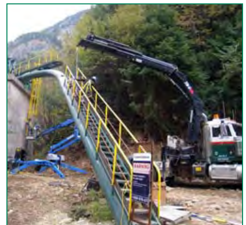
Stairs, prior to being removed from the pipeline
