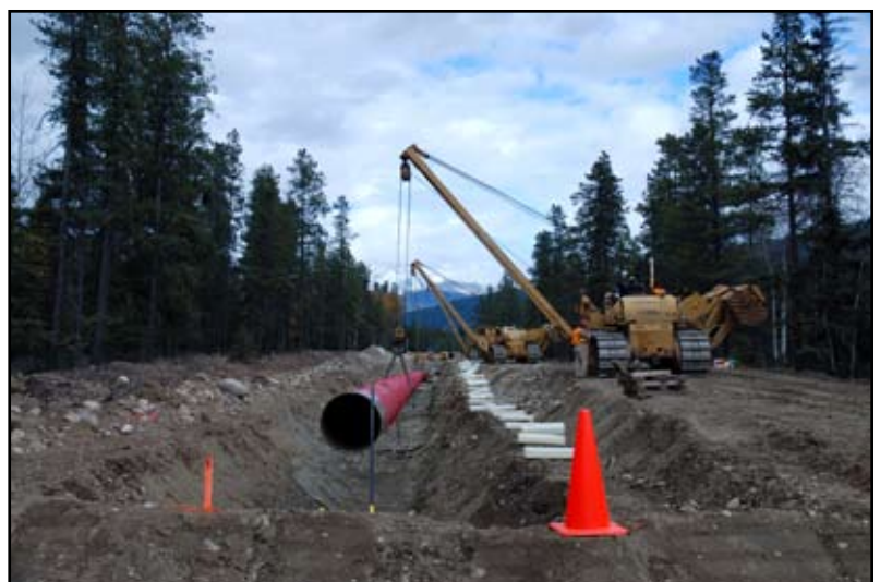
Lowering pipe into ditch, Jasper, Alberta
